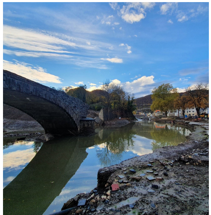
Evidence of devastation in most of the villages along the Ahr River, Germany, is still present – including in Altenahr, even four months after the July flood event. (Source: RMS, November 2, 2021)
