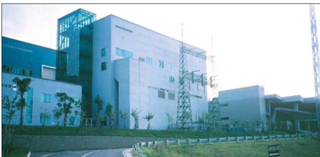
The newly-opened cogeneration plant is an independent power producer and a valuable auxiliary power source for several semiconductor businesses in the Hsinchu Science Park.
