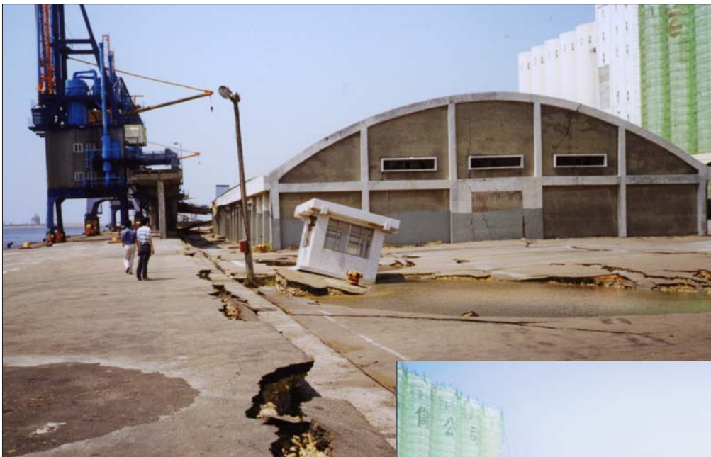
As much as four feet of ground settlement was observed along the entire length of a wharf (approximately 1,000 meters, or 3,300 feet) at the port of Taichung.
