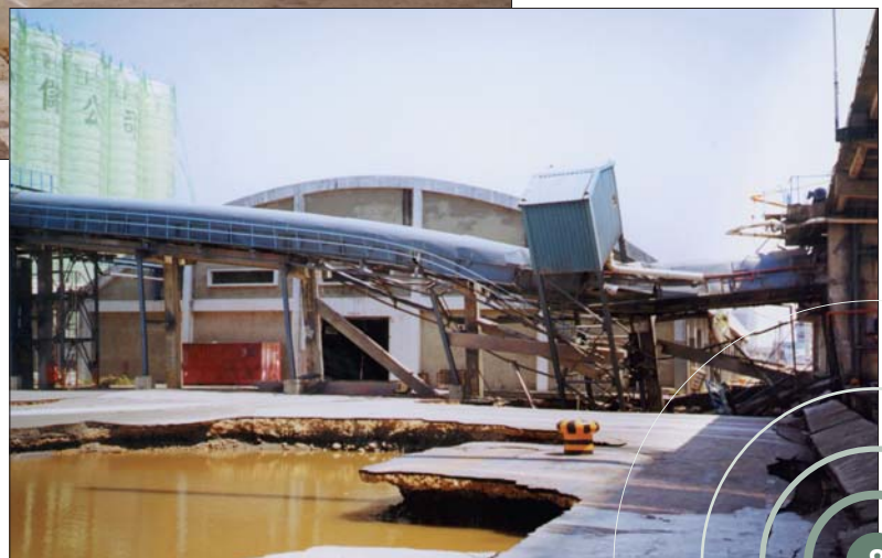
As much as four feet of ground settlement was observed along the entire length of a wharf (approximately 1,000 meters, or 3,300 feet) at the port of Taichung.
