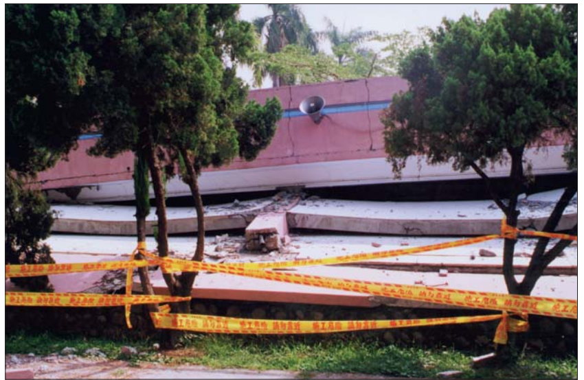
A pancaked classroom building on a junior high school campus in Wufeng.
